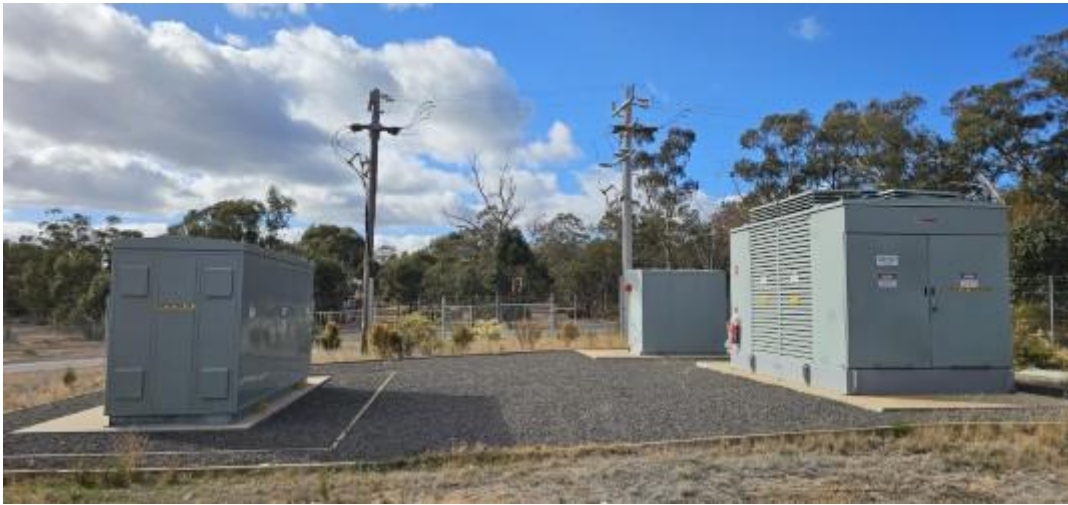
Photo 1: Powercor supply poles, sub station 1, REFCL isolation transformer 1;1
