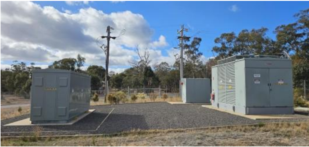
Figure 2 Powercor supply poles sub station 1 with REFCL Isolation transformer 1
